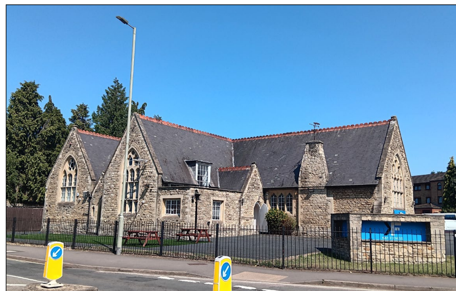
St Leonards Primary School Building
